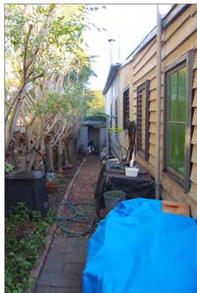
Figure 11: Eastern side of the dwelling, looking south, showing the rear skillion.
