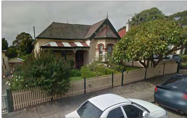
Figure 40: 68 Prospect Road, Summer Hill. Locally listed item. Google Maps, 2016.
