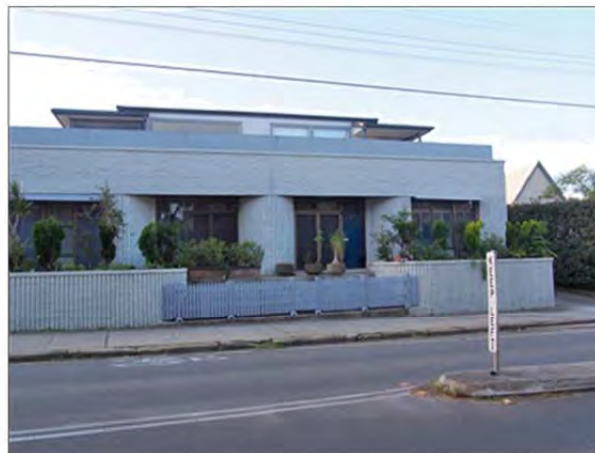
Figure 33: Nos. 41-43 Smith Street, adjoining the site to the west.
