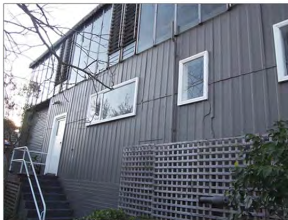
Figure 29: Details of the southern elevation.
