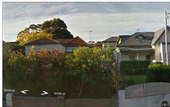
Figure 34: Nos. 33-35 Smith Street, adjoining the site to the east. Google Maps.
