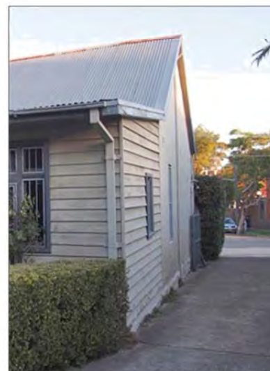
Figure 13: Western elevation of the dwelling, looking south.
