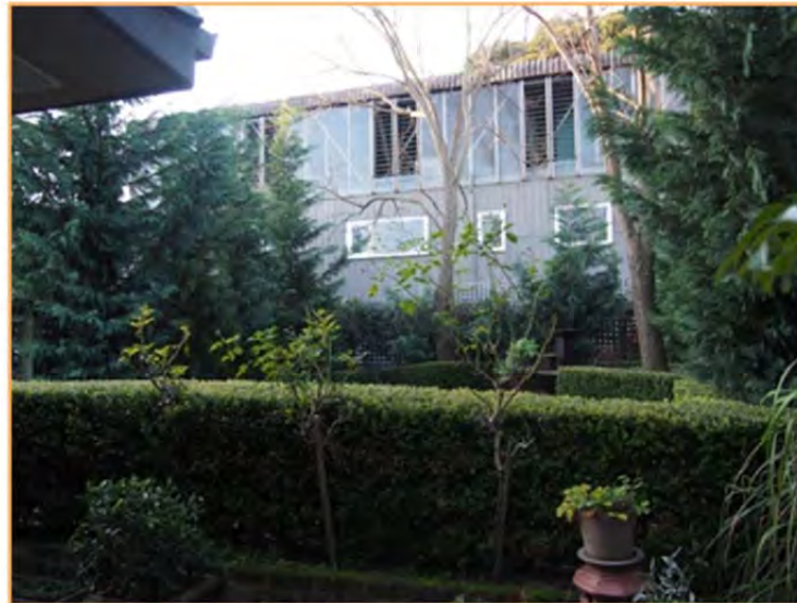
Figure 3 – view of factory at rear of site (Source: Heritage Report, Weir Philips)
