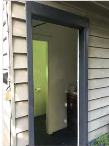
Figure 27: Fibro lining and external bathroom fit out.
